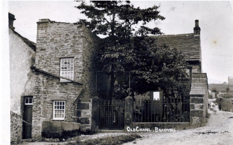
Chapel in Charlotte Lane top of Smithy Hill
